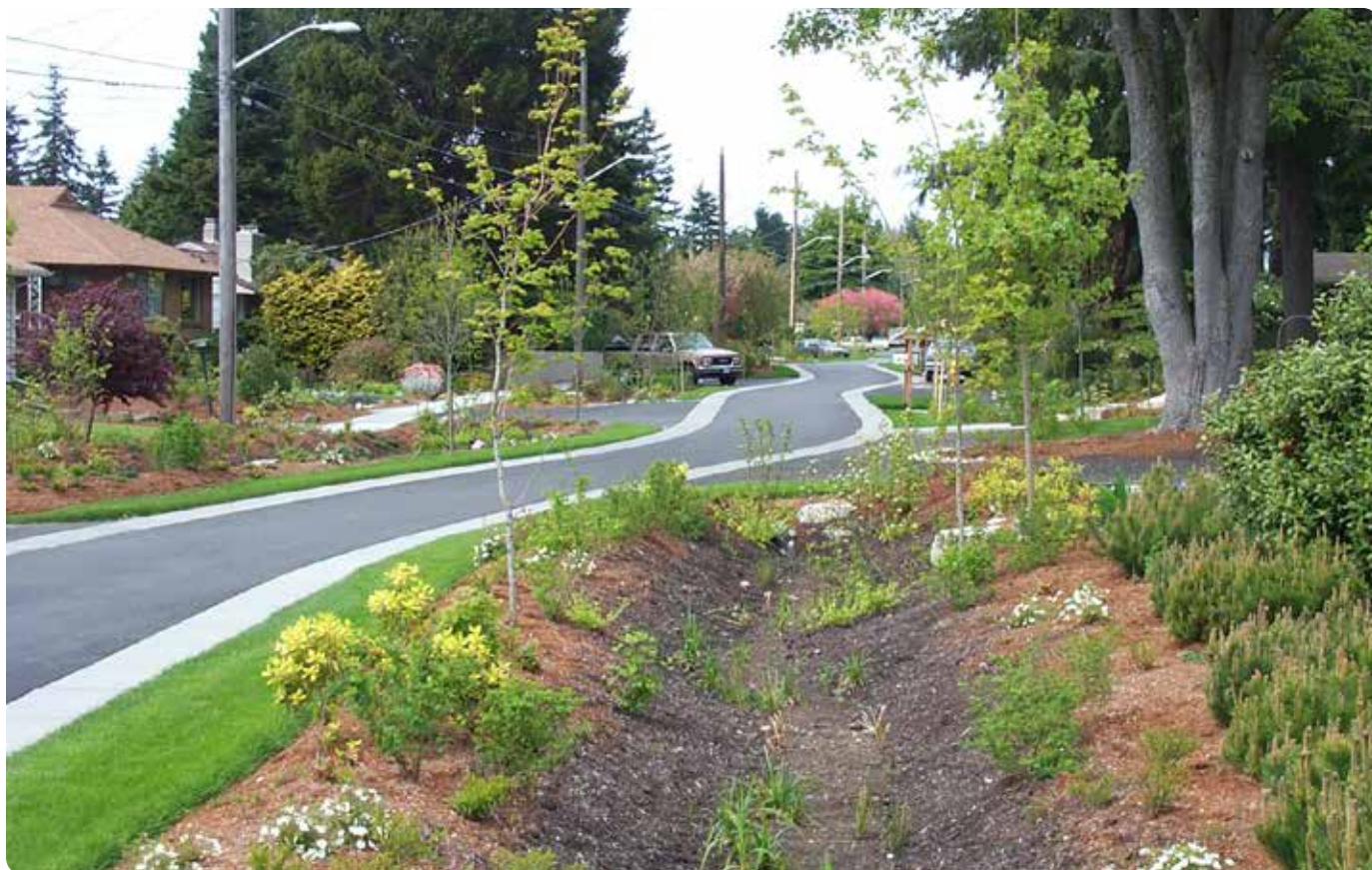
▲ GREEN STREET EXAMPLE SHOWING BIORETENTION AREAS AS A PART OF THE STREETSCAPE
